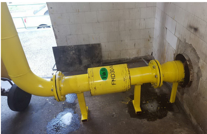
Sample Horizontal Installation FHD30-NG In Line
