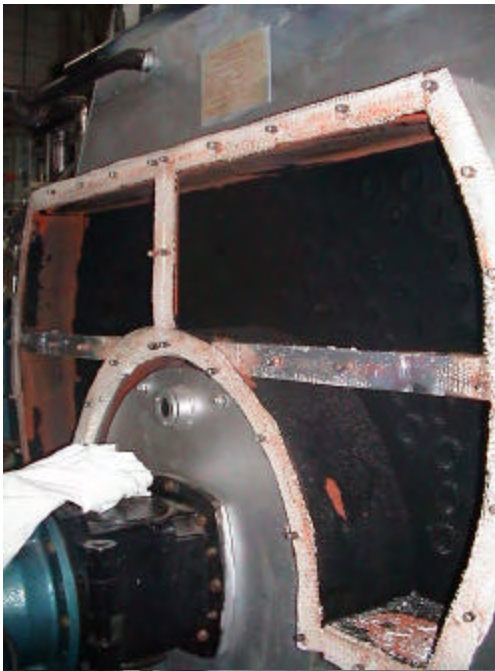
Tube Condition Before Installation
