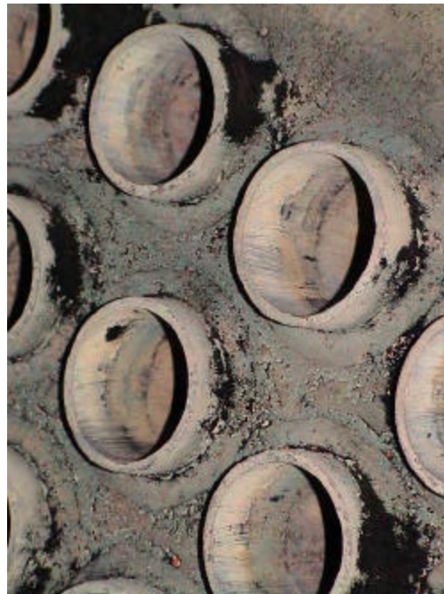
Tube Condition After Installation
